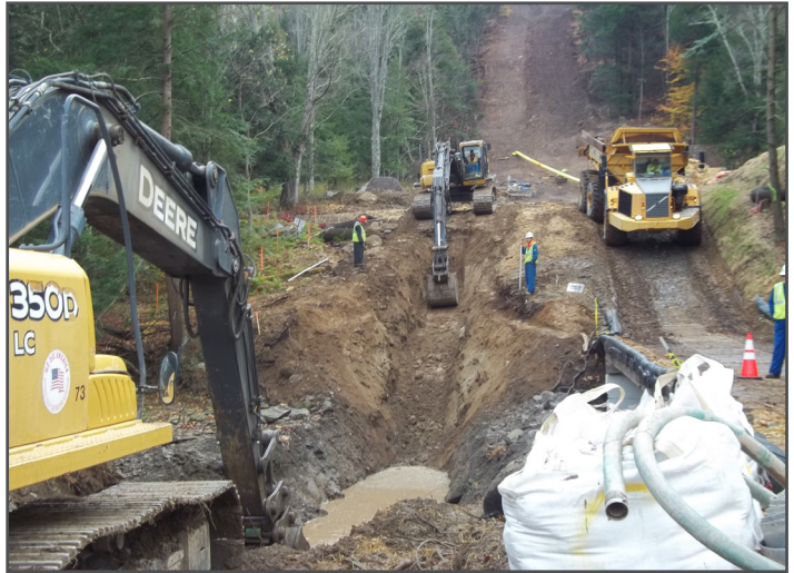
Image of stream crossing from www.lindeco.com
