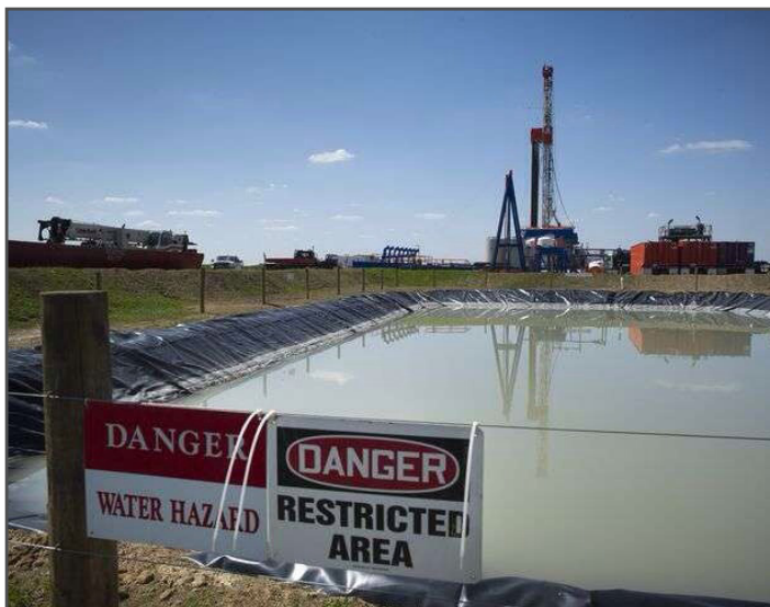
This is a hydraulic fracking wastewater pit used to store waste until it is transported by pipe or truck to a disposal site. The US Coast Guard is considering options for allowing this toxic soup to travel on our national waterways.
