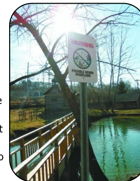
"WARNING: Possible sewer overflows." The City of Bardstown was forced to place signs along Town Creek by the state's Dept for Environmental Protection's Division of Enforcement.
