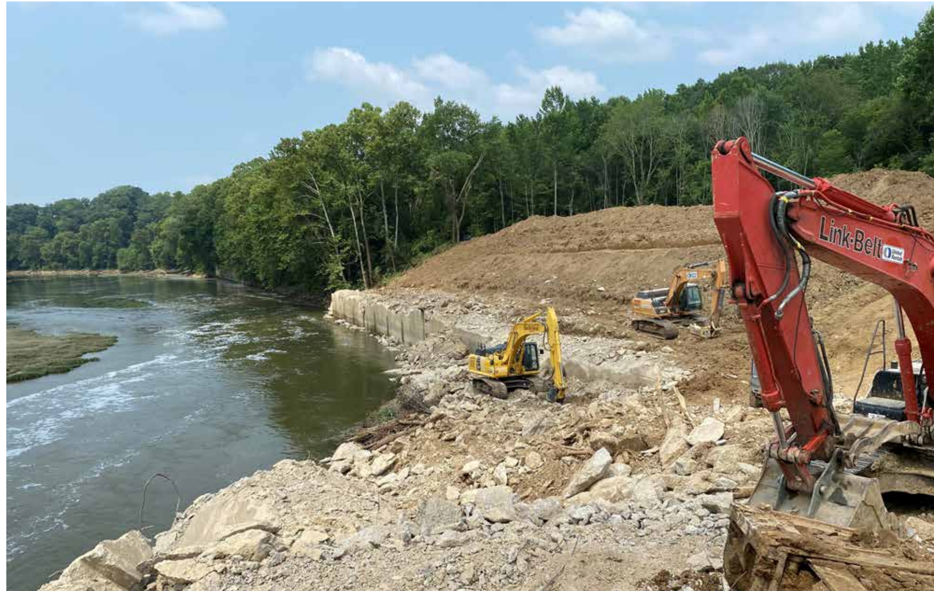
Demolition of lock chamber, looking downstream
