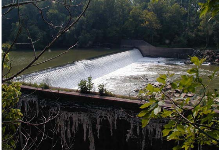
Green River Lock and Dam 5
