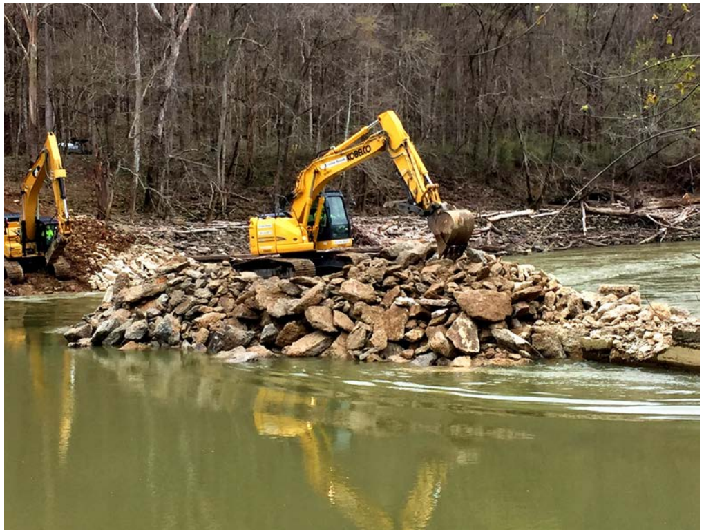
Green River Dam 6 demolition 2017
