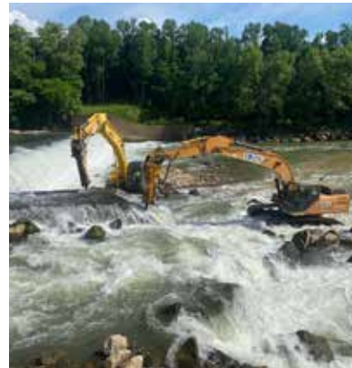
Contractors demolishing Green River Dam 5
