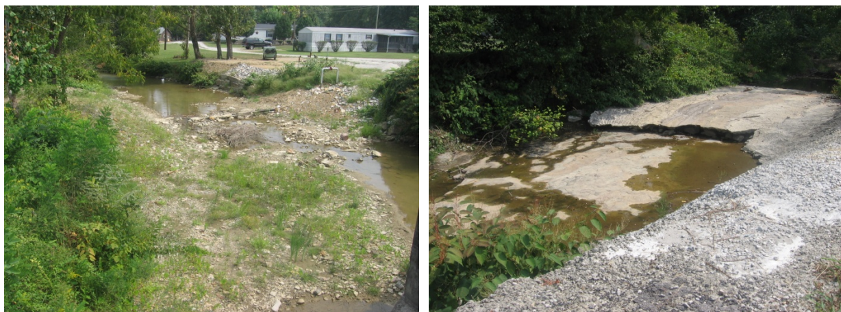
Figure 3.6. Examples of pipeline crossings on Dry Creek.
