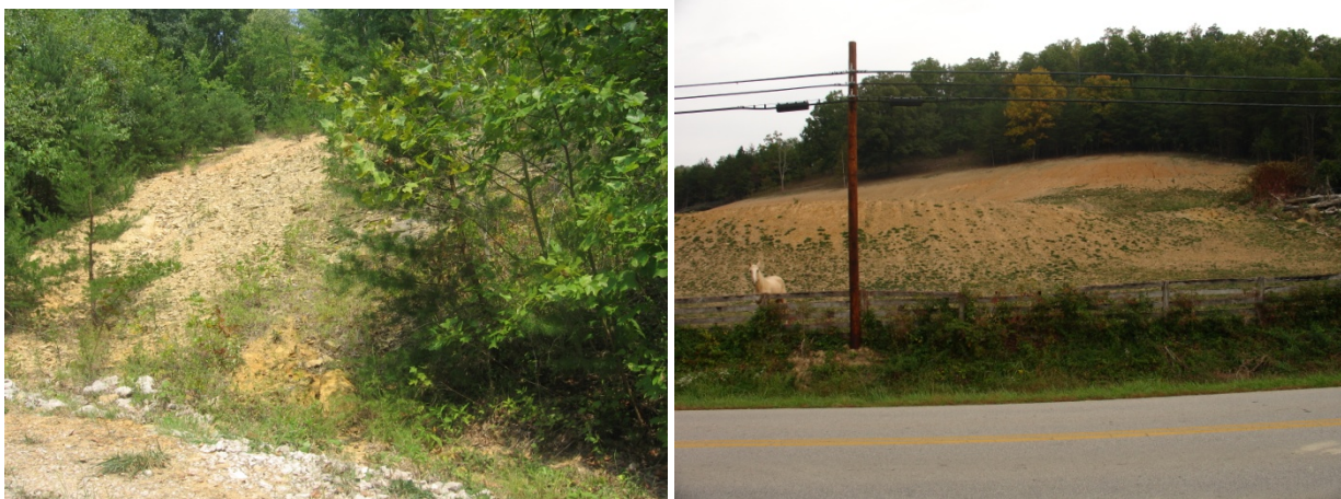
Figure 3.5. Example of vegetative cover being removed and not replanted.
