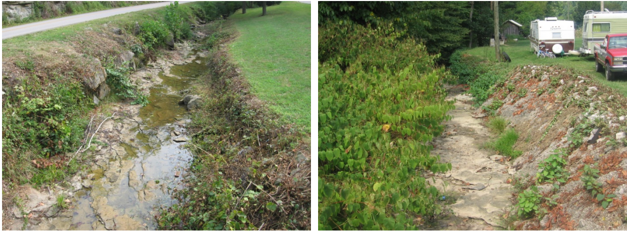
Figure 3.7. Examples of stream straightening and private bank armoring.
