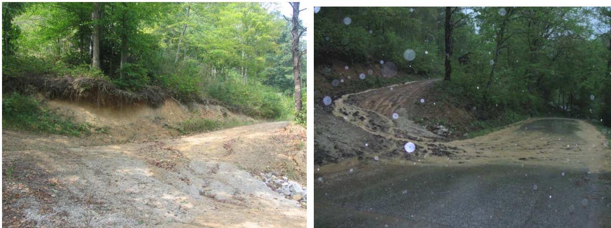
Figure 3.8. An example of poor land use. The photo on the left is a road cut into a hillside. Note the overhanging, eroded bank and gullied road. The photo on the right is the same site during moderate rainfall.
