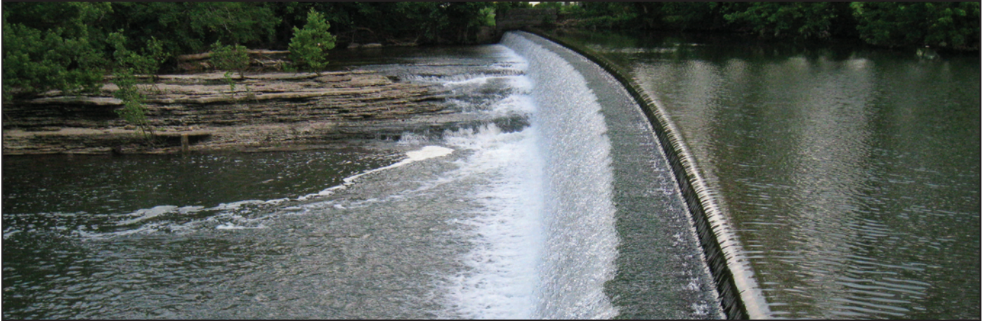
Low-head dam on South Elkhorn Creek
