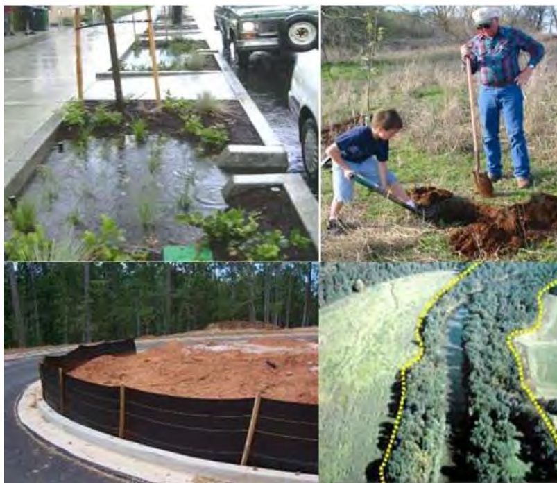
Figure 5.1: Examples of structural best management practices.
